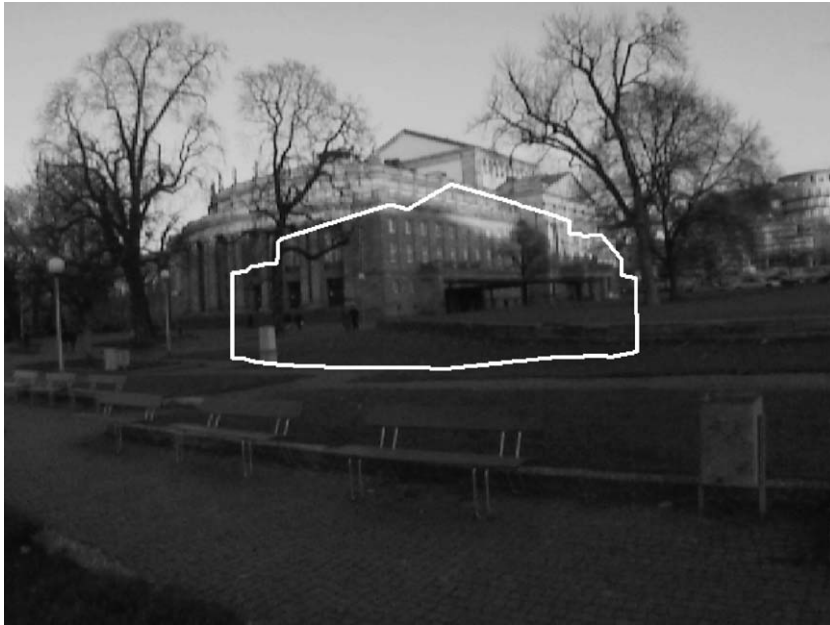
Fig. 2. Silhouette of the building as projected to the image based on the exterior orientation from GPS and digital compass.
